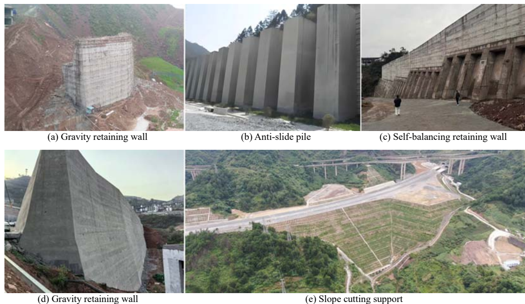
Fig.1 Typical retaining structures for high fill slopes
