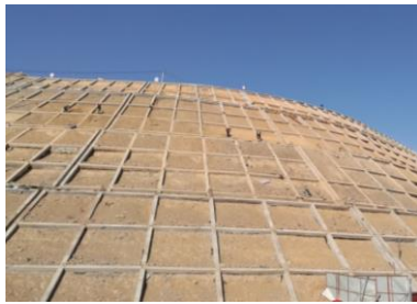
Fig. 10 A slope supported by frame anchor plates
