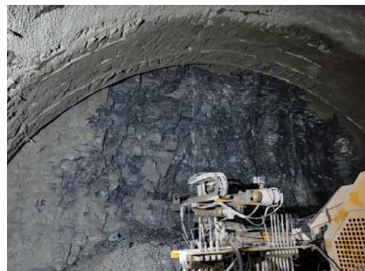
Fig. 1 Tunnel face for in situ digital drilling test
