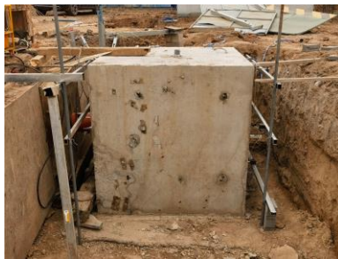
(b) Single pile cap
