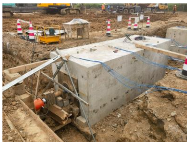
(c) Double pile cap
