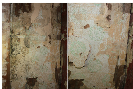
Fig. 18 Patterned wallpaper on the back wall of Tishun Tang in Yangxin Dian
