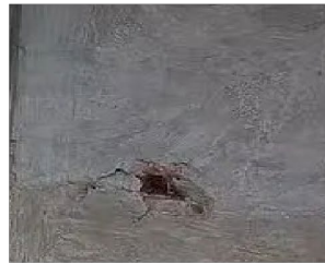
(b) Exposed reinforcement
