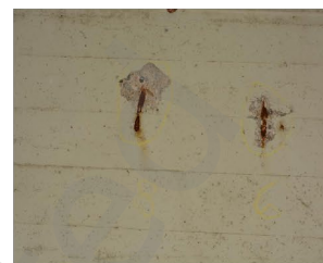
(b) Exposed reinforcement
