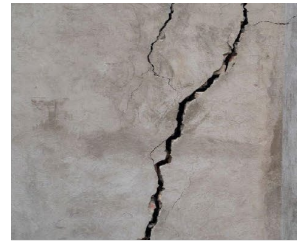
(a) Concrete crack
