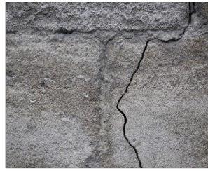
(a) Concrete crack
