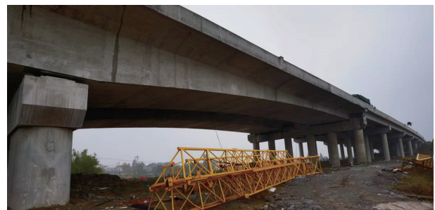
Fig. 1 Actual photo of the South span of the tested bridge. Photograph by Yu Zhou 2023.
