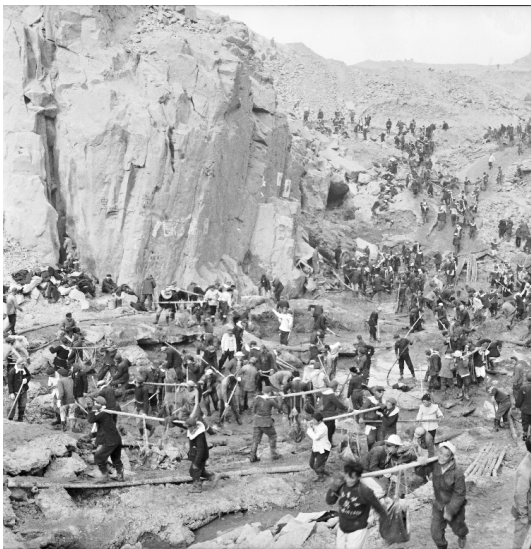
Fig. 5 Sediment removal in foundation pit (provided by Sinohydro Bureau 11 Co., Ltd.).
