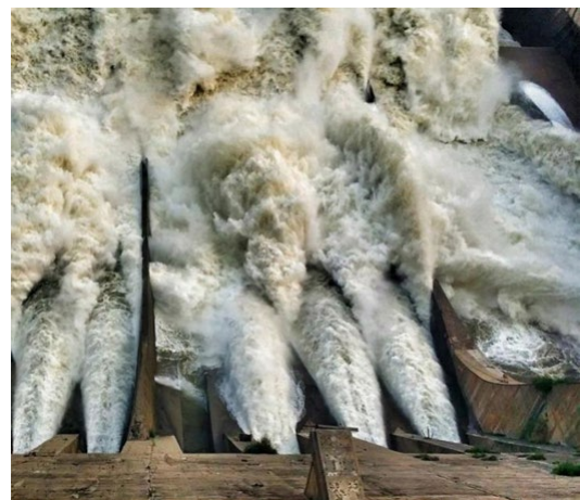
Fig. 9 Discharge view of Sanmenxia hydro-junction.
