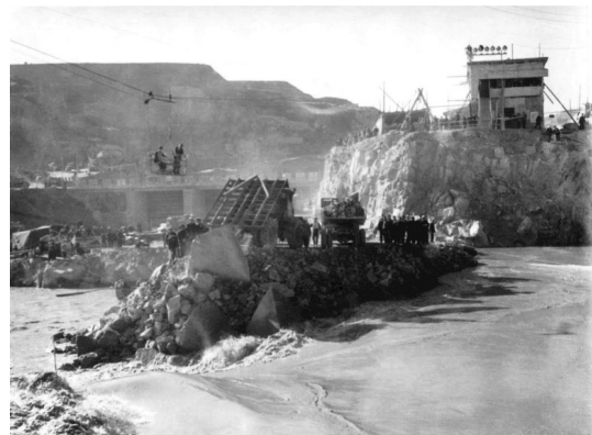
Fig. 4 River cutoff for foundation pit (provided by Sinohydro Bureau 11 Co., Ltd.).
