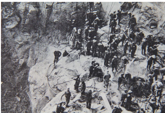
Fig. 6 Rock excavation for dam foundation (provided by Sinohydro Bureau 11 Co., Ltd.).
