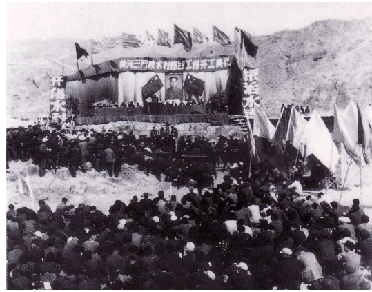
Fig. 3 Commencement ceremony of Sanmenxia hydro-junction (provided by Sinohydro Bureau 11 Co., Ltd.).
