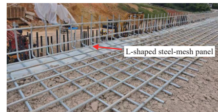
Fig. 2 L-shaped steel-mesh panels used as temporary facing.
