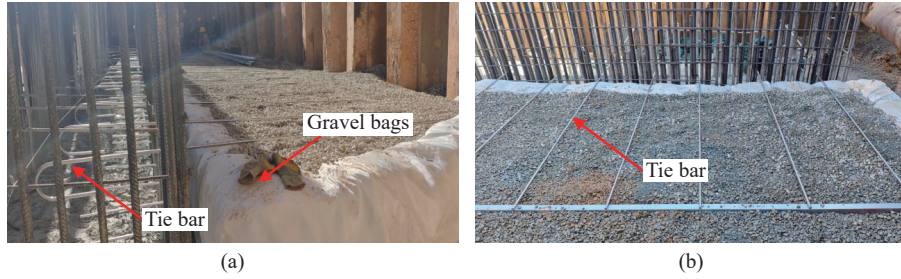
Fig. 4 Construction of tie bars. (a) Side view; (b) Top view.
