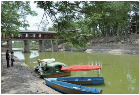
Fig. 5 A pedestrian stone-beam covered bridge as a viewpoint for the Zhaozhou Bridge.
