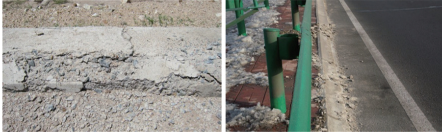
Fig. 1 Curb corrosion
