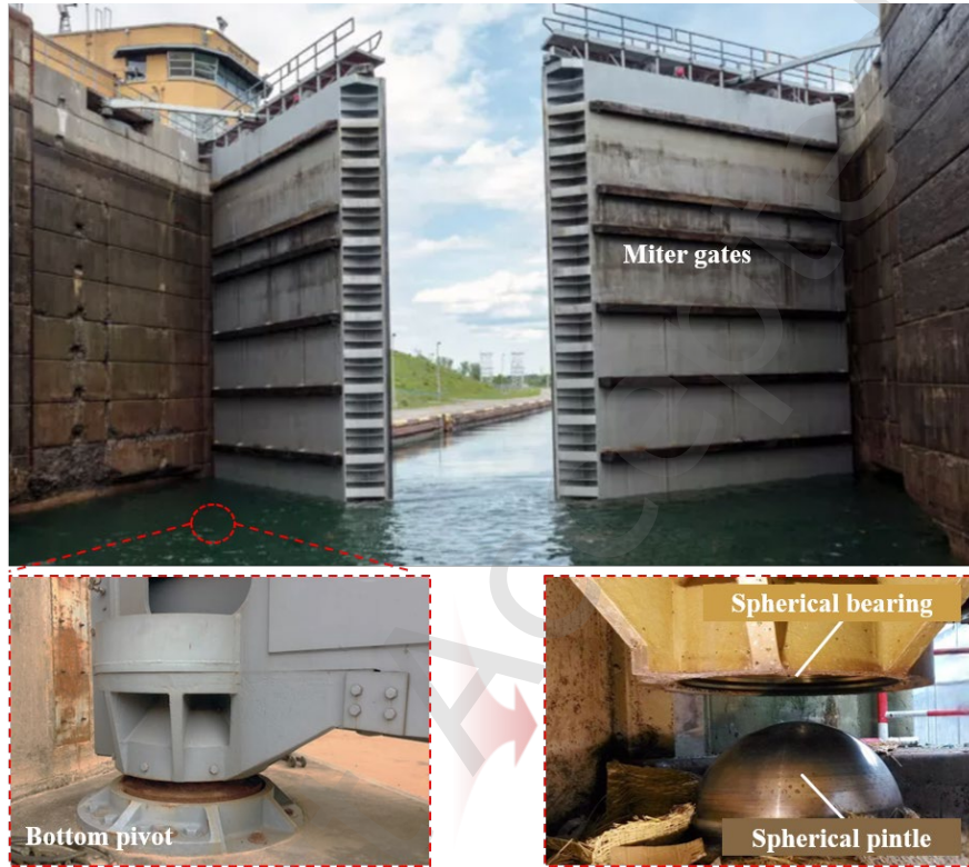
Fig. 1 Schematic diagram of the bottom pivot friction pair of miter gates.
