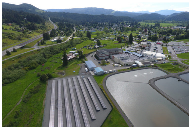
Fig. 4 Overview of the BLR community microgrid (Source: Schatz Energy Research Center, Humboldt State University) [31] .
